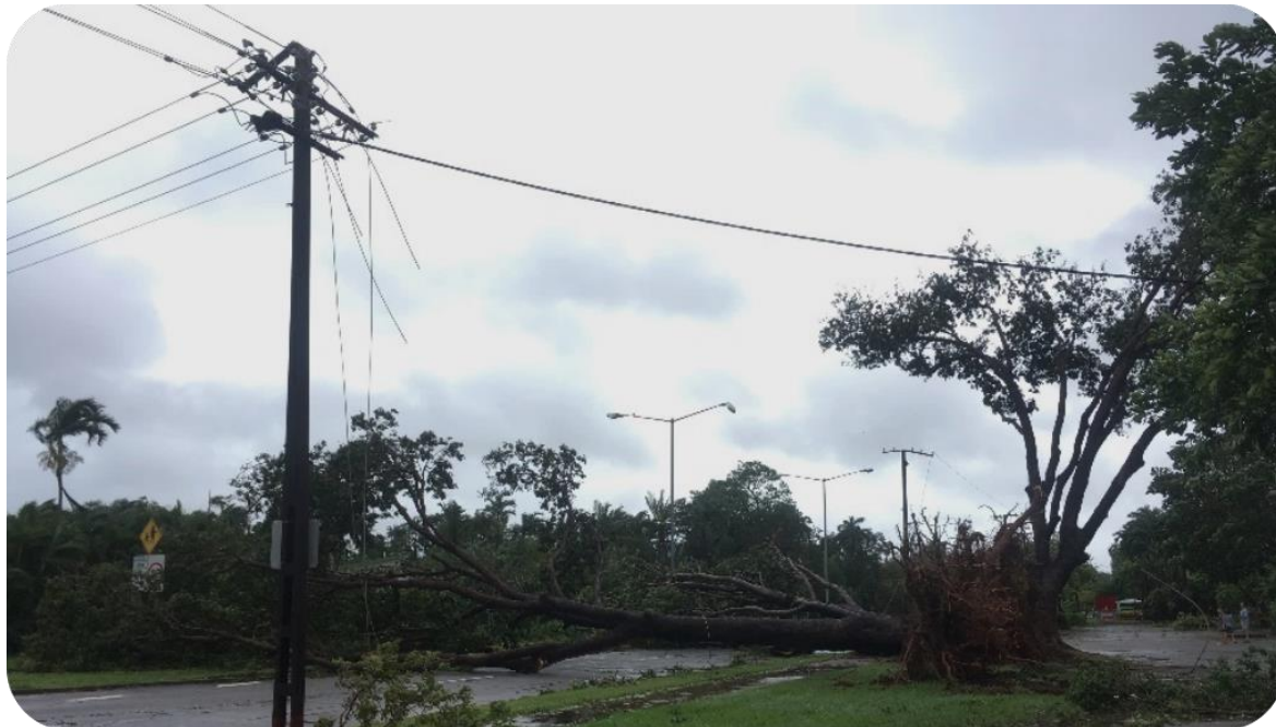
Figure 6-2: Storm damage to electrical transmission lines.
